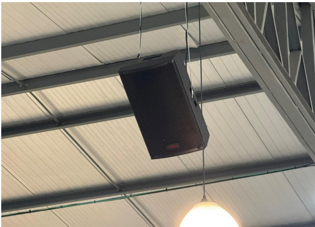
Figura 10 - Point Source Suspenso
